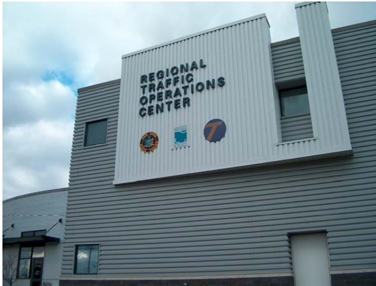
Figure 1-1. Rochester N.Y. Regional Traffic Operations Center.
