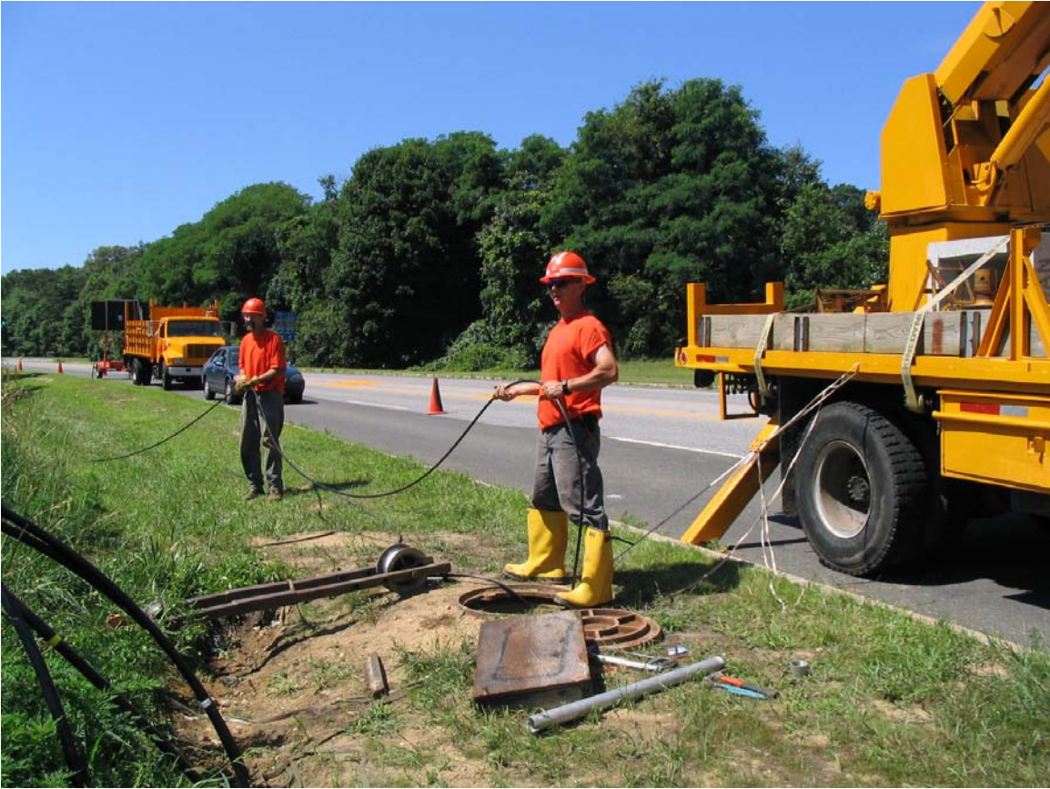
Figure 9-1. Installing Communications Cable.
